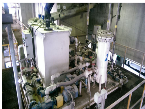
Fig. 3. Ball mill lubrication system
