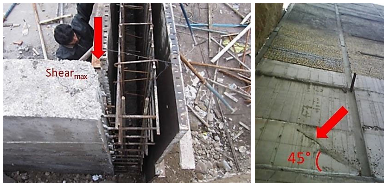
Fig. 3. Wrong construction joint position at a concrete wall joint (left) and a shear wall (right)
