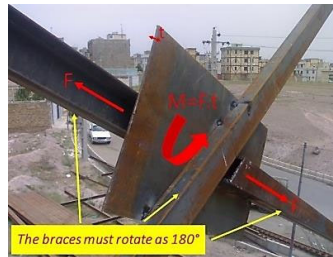
Fig. 8. An example of structural issues due to construction errors in the bracing system
