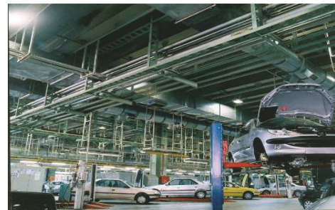
Fig. 13. The image of the project after completion
