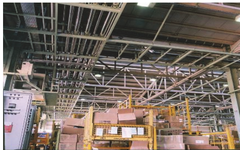
Fig. 12. Image of the Piping activitie
